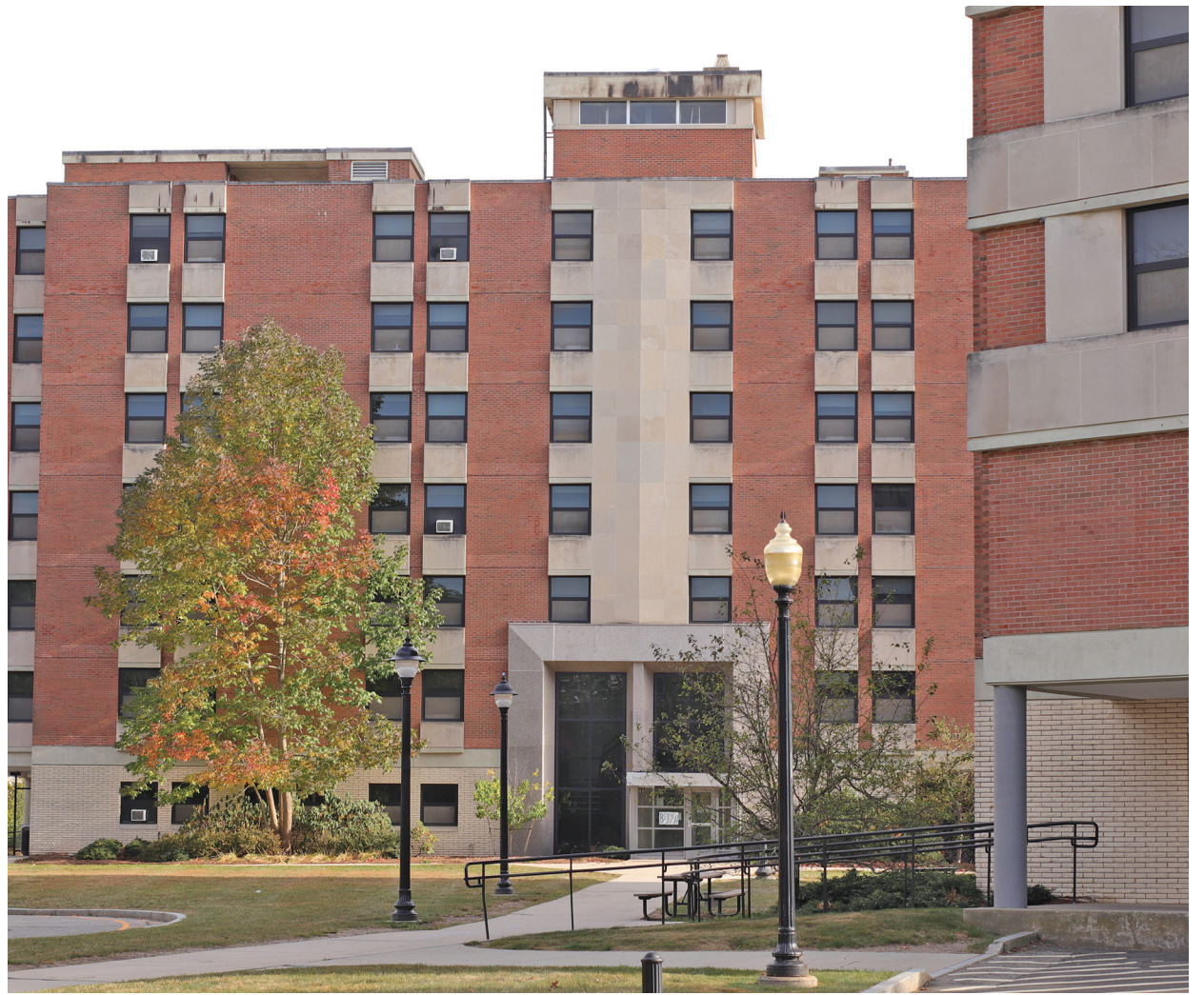
L. Richard Belden Hall, in the Alumni residential quad on the Storrs campus. Alumni, along with the West quad, were the last building to regain power during the March 21, 2022 outage. PHOTO BY ERIN KNAPP, ASSOCIATE PHOTO EDITOR/THE DAILY CAMPUS
