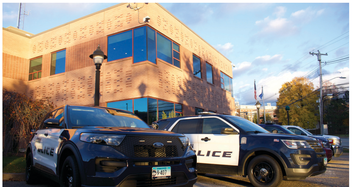
The University of Connecticut's Police Department, renamed the “Public Safety Complex,” sits down the hill from Northwest dorms. This houses UConn's Fire, EMS, and Police departments that service UConn and the nearby community. FILE PHOTO/THE DAILY CAMPUS
