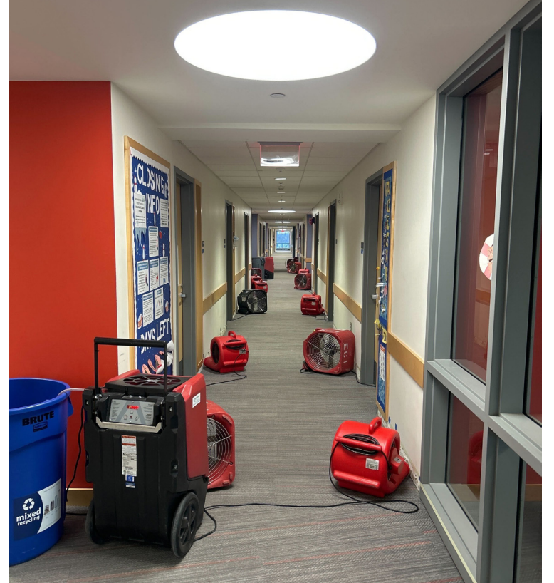
Sprinklers were activated on Tuesday, Nov. 28, 2023 in Peter J. Werth Tower due to high heat being detected in a residential room. University Safety responded to the situation and two people have been arrested. PHOTO BY TOMAS HINCKLEY, GRAB PHOTOGRAPHER/THE DAILY CAMPUS
