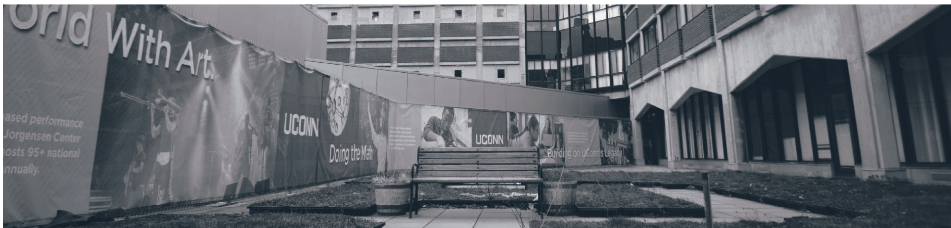
Construction continues this semester on the Gant Science Complex, expanding across the elevated platform. PHOTO BY AVERY BIKERMAN, GRAB PHOTOGRAPHER/THE DAILY CAMPUS
