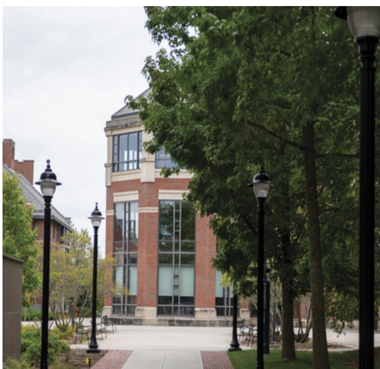
UConn's South Campus in Storrs, Conn. South Campus' geothermal power project is set to be completed in February 2026.
