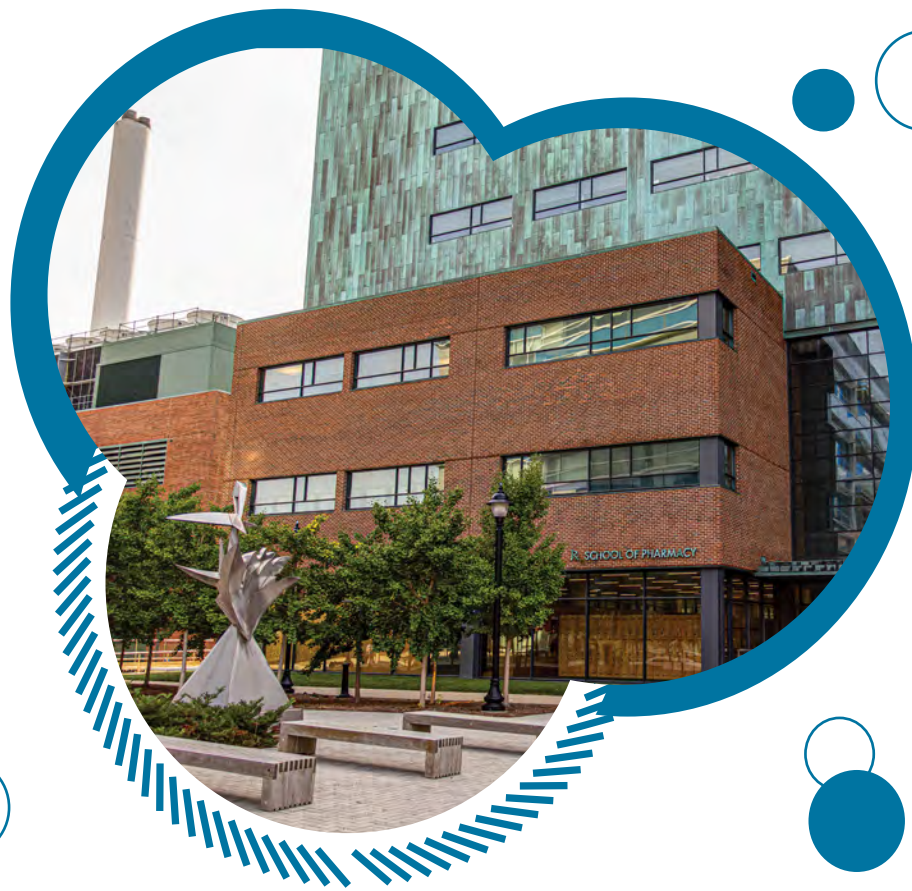
Exterior of the University of Connecticut School of Pharmacy on the Storrs campus. The main entrance features a modern design combining brick, a glass atrium and a patinated copper facade. PHOTO BY PARKER MEYERS, GRAB PHOTOGRAPHER/THE DAILY CAMPUS
